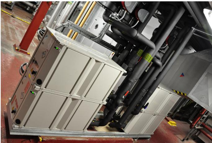
primary cooling for the data centre - reducing the return flow temperature in the existing circuits from 12°C to 9.5°C. The heat pumps then enhance the rejected heat through their refrigerant circuits before transferring it to the AHUs via secondary water circuits. DCI's clever plumbing enabled the groups of Daikin units to tap into the existing water circuits, and to serve the three AHUs.
